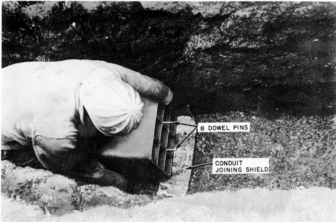
Fig. 15-31 - Placing 9-Duct Multiple Tile Conduit
