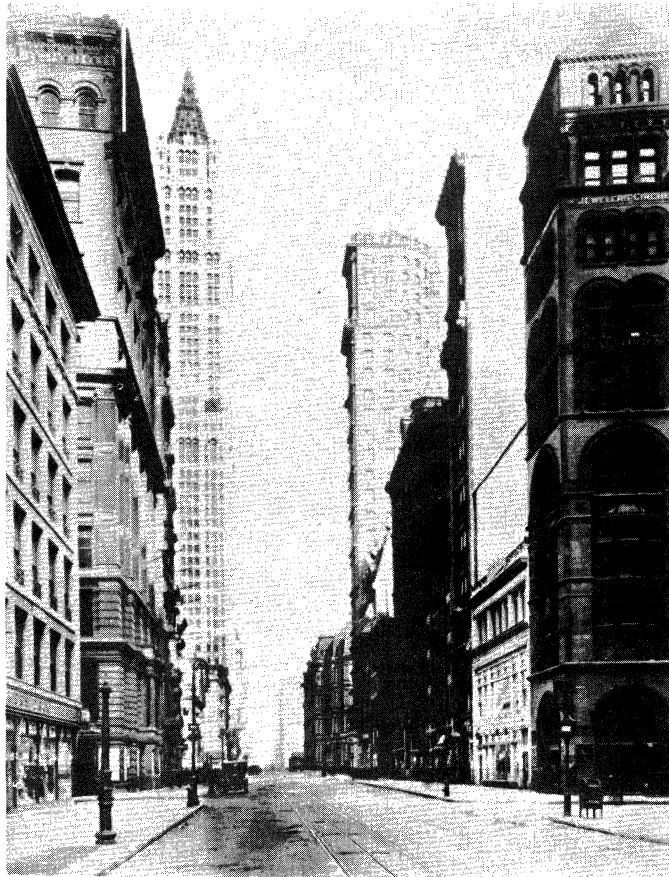
Fig. 15-4 — Lower Broadway, New York, After Underground Facilities Were Installed
