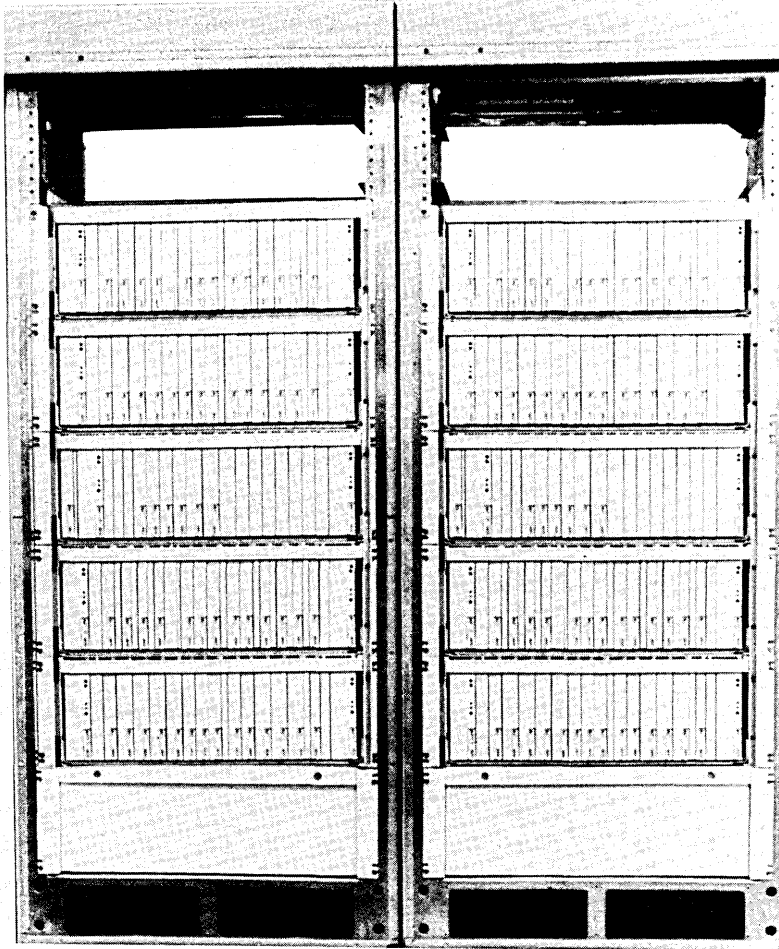
Fig. 17—Time-multiplexed switch cabinet.
