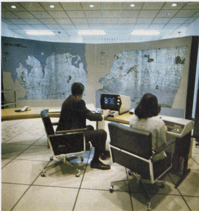
Displays of computer-controlled-traffic data plug operators into LFE's system. Their inputs and overrides are fed to the central processor by means of English-language instructions, in this 5000 series system.
