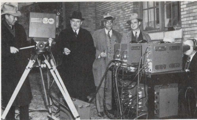
1939—The first godfather? Nope. Chairman J.L. Fly and members of the FCC inspect newly developed, "light-weight portable" field equipment, weighing one-tenth that of the only other available unit.
