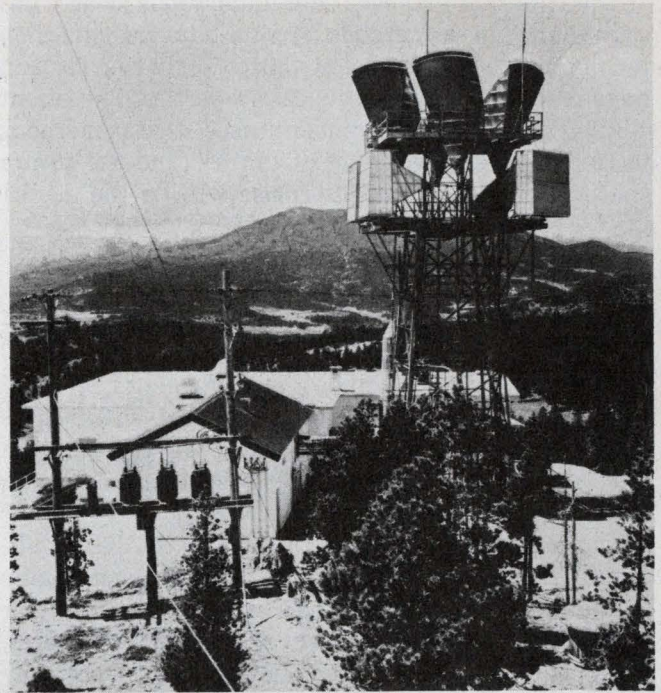
1960—Radio-relay stations like this Western Electric TH microwave system between the Denver-to-Salt-Lake-City route standing atop Buckhorn Mountain (8306 ft) in Colorado, start taking over from cables and lines.
