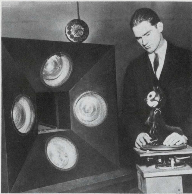
1928—America's first television star , a blurry Felix the Cat, whizzed from RCA studios in Manhattan to awe the folks in Kansas, in tests of early pickup devices and primitive 60-line receivers.
