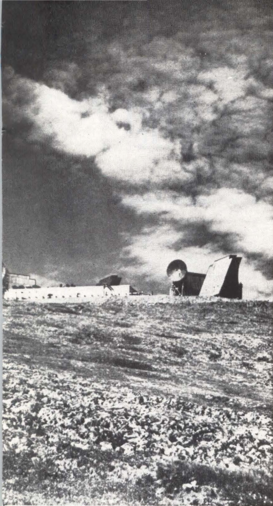
ALASKAN SWITCHING system built by Western Electric provides direct dialing without private line and manual switchboards. DCA wants USAF system modified to handle Army, Navy, and FAA
