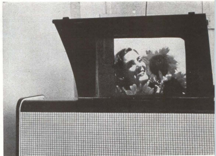
Experimental model of banana-tube system displaying a color picture
