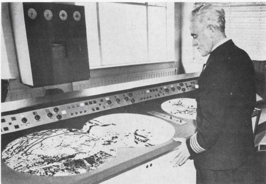
Two for Tees. Harbormaster can check movements of all ships in Tees estuary on display that puts data from pair of overlapping radars onto a projected chart.
