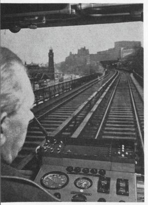
On the track. Siemens control system is under test for the Hamburg subway.
