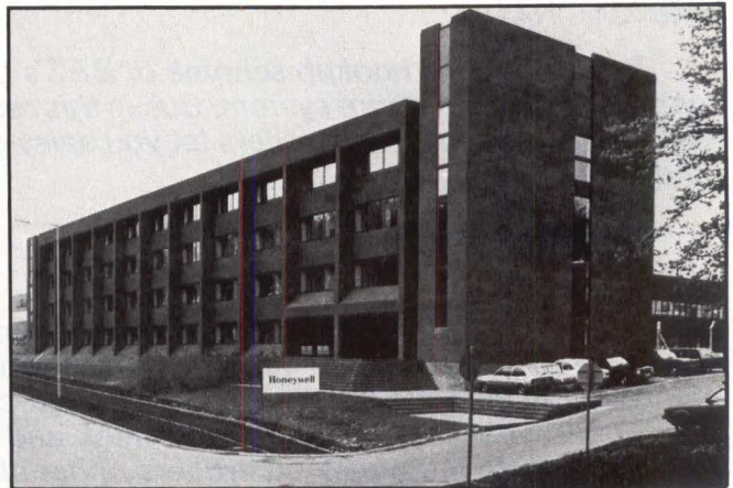
Honeywell Information Systems Ltd.'s 112,000-sq.-ft. headquarters in Hemel Hempstead houses a software group that conceived, designed and produced the company's TPS-6 transaction-processing system.
