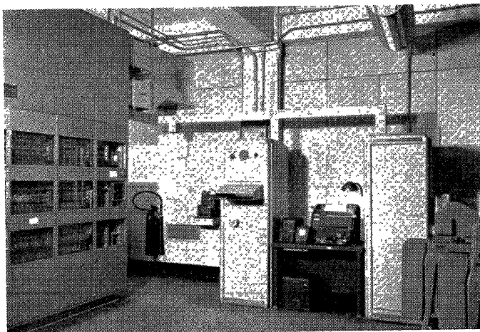
Figure 3 (left). ORDVAC with perforated tape-handling device in central background, and card-handling equipment at extreme right
