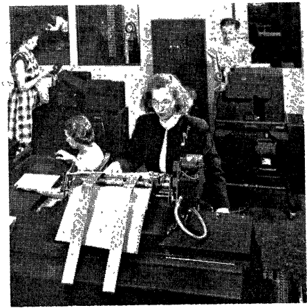
Figure 4. Card and tabulating equipment associated with ENIAC at Aberdeen Proving Ground
