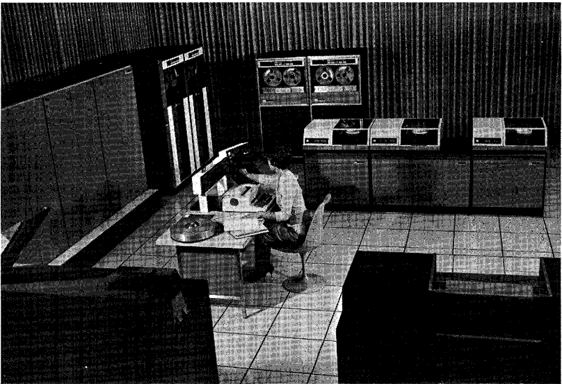
Fig. 6-1. A Computer Installation. (Courtesy, Data Processing Division, International Business Machines Corporation)
