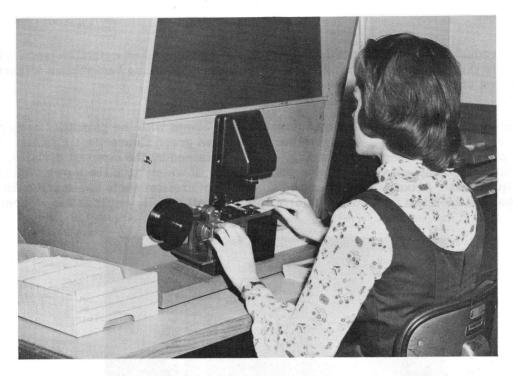
APERTURE CARD MOUNTER permits microfilm pictures of engineering tracings to be mounted in preprinted aperture cards.
