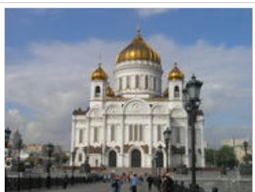
Cathedral of Christ the Saviour, demolished during the Soviet period, was reconstructed from 1990–2000
