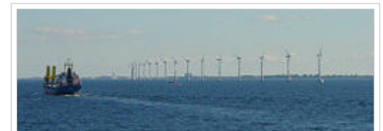
Offshore wind turbines near Copenhagen
