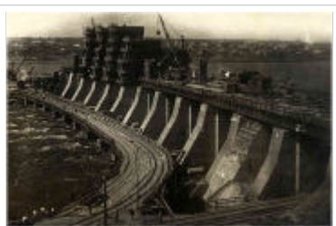
DniproGES hydroelectric power plant under construction circa 1930
