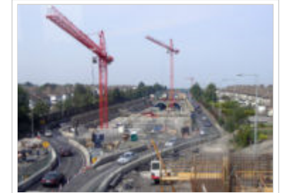
Dublin Port Tunnel under construction.
