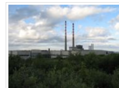
Ringsend power station, Dublin.
