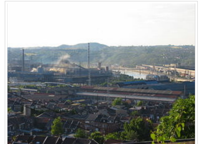
Steelmaking along the Meuse River at Ougrée, near Liège
