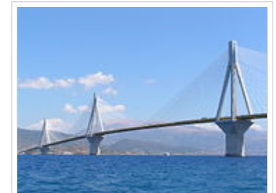
The Rio-Antirio bridge near the city of Patras is the longest cable-stayed bridge in Europe and second in the world. It connects the Peloponnese with mainland Greece.
