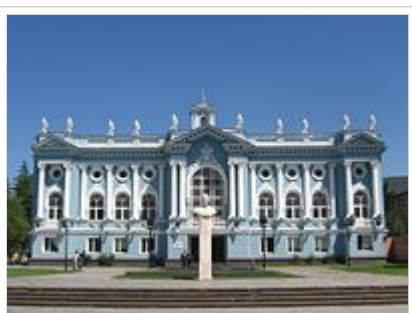
Akaki Khorava State Theatre in Senaki, an example of neoclassicism style with elements of barocco in Georgia. Architect Vakhtang Gogoladze.
