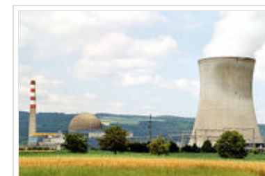
The Leibstadt Nuclear Power Plant is located in the canton of Aargau.
