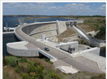
Alqueva Dam, Alentejo - irrigation and hydroelectric power generation facility which created the largest artificial lake in Western Europe.
