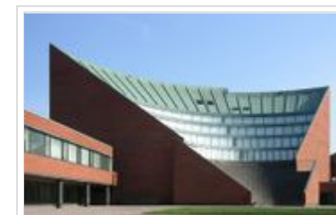
Auditorium in the Helsinki University of Technology's main building, designed by Alvar Aalto.
