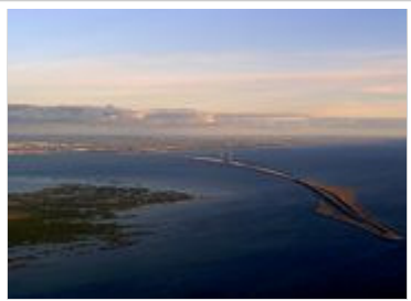
Øresund Bridge from Denmark to Sweden. On the right is the artificial Peberholm island, and on the left Saltholm. Picture is taken from the air.
