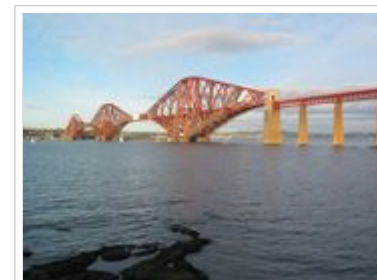
The Forth Bridge, Scotland: an iconic feature of the rail network
