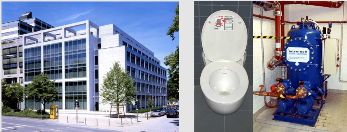
Figure 19: KfW office building “Ostarkade” (left); Vacuum toilet and pumping unit (right) (KfW)
