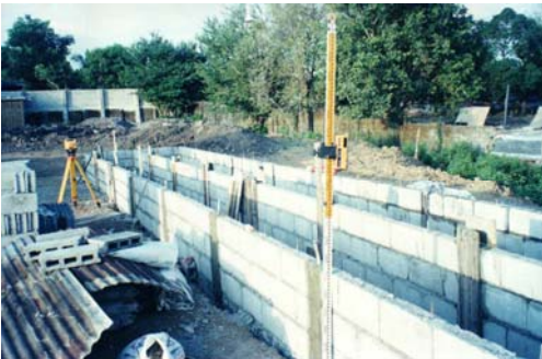
Figure 3-2 Laser-level equipment used to ensure proper elevations during construction.
