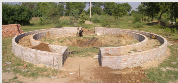
Figure 32: Urine-separation vermi composting toilet (left) and new school toilet block with bio-gas treatment - under construction (right). (GTZ)
