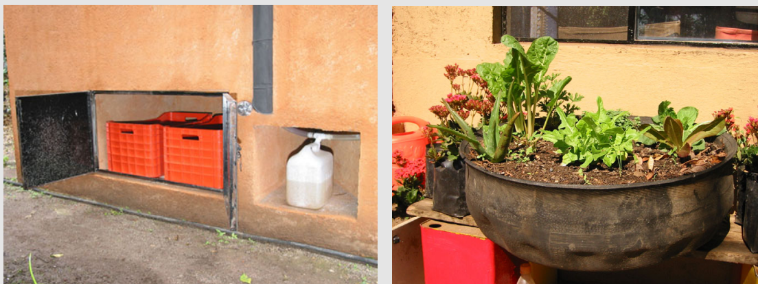
Figure 9: Dehydrating chamber with 2 containers and urine collection (left); organoponics (right) (TepozEco)
