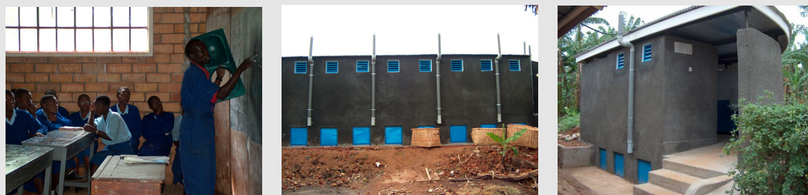
Figure 22: Training of students (left); dry toilets with wooden containers for collecting the separated faecal material (middle - view from the back) and demonstration toilet (right). (EcoSan Club)
