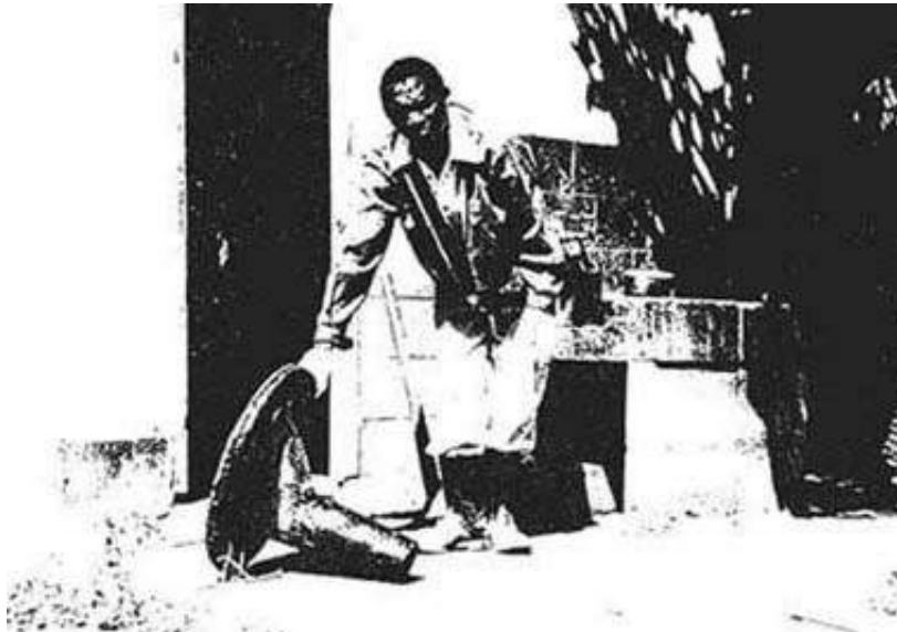
Photograph 9: Cast iron squatting plate with integral drop pipe, fitted in a toilet block with interceptor tank below. The squatting plate is removed to empty the tank
