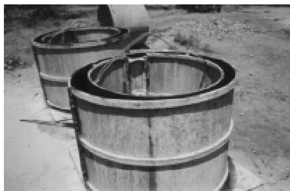
Photograph 11-2 - Formwork assembled and ready for use
