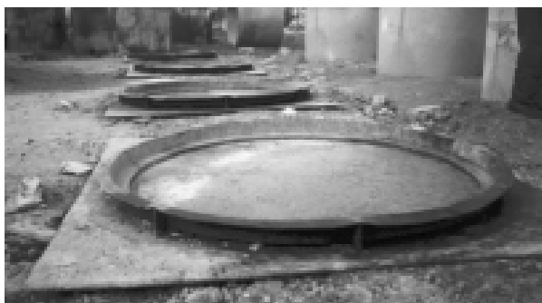
Photograph 11-8 - Rebate rings in position, awaiting assembly of formwork
