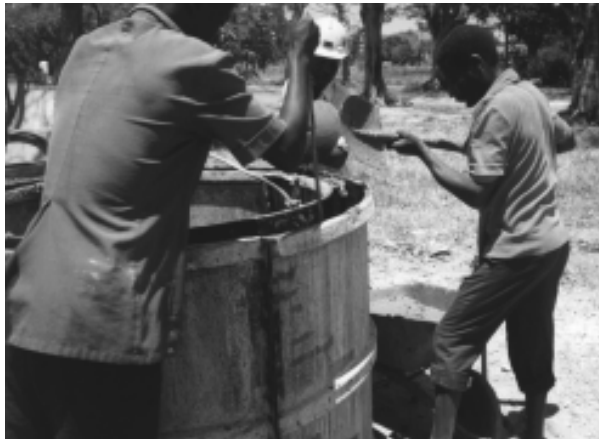
Photograph 11-4 - Rodding to ensure compaction
