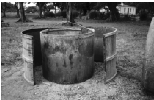
Photograph 11-1 - Inner and outer formwork, dismantled
