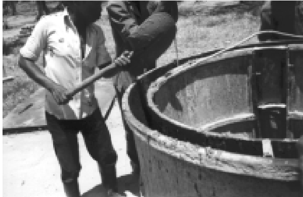
Photograph 11-3 - Pouring a ring
