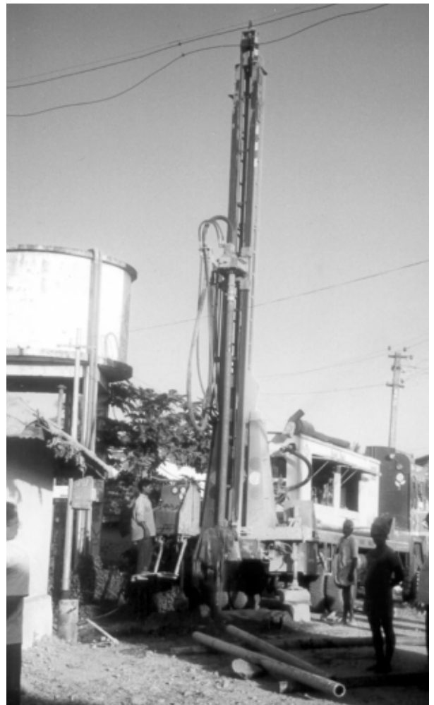
Photograph 4-2 - A rotary drilling rig
