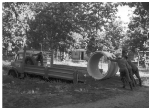
Photograph 11-6 - Loading a concrete ring using a temporary loading ramp
