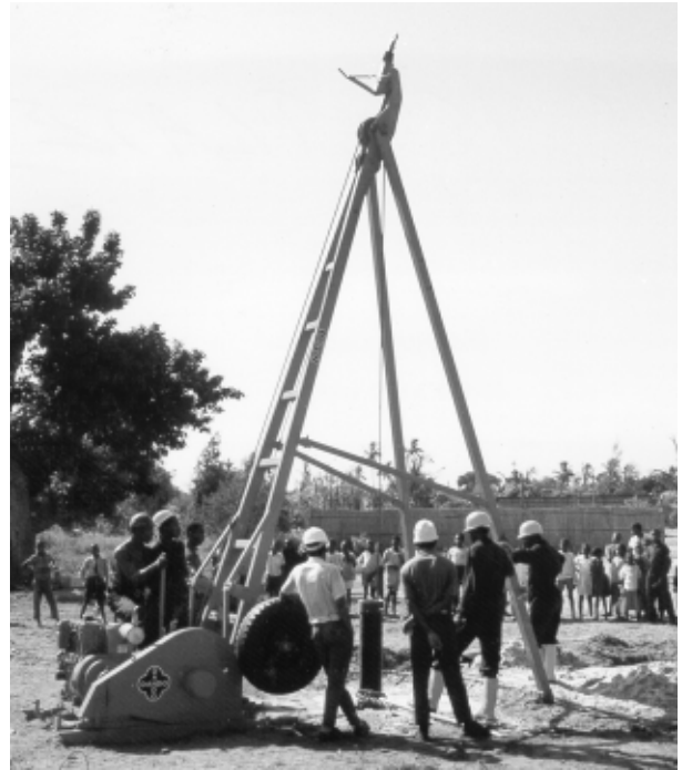
Photograph 4-1 - A percussion drilling rig
