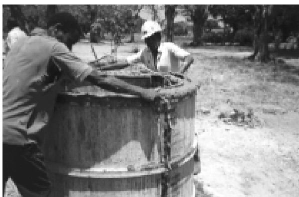
Photograph 11-5 - Finishing off at the top of a ring
