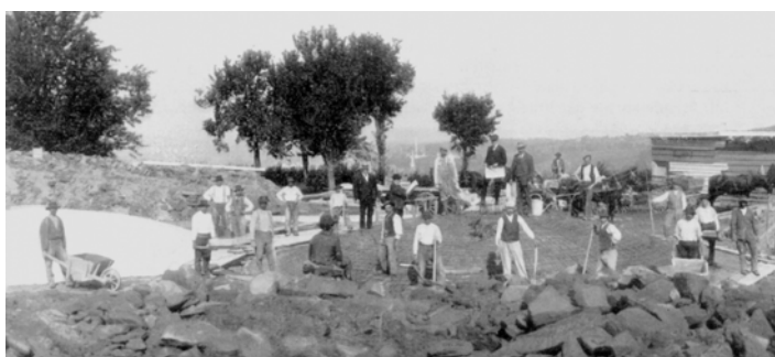
Photo 7 Community involvement in the construction of a reservoir over 100 years ago
