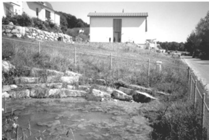
A larger retention pond serving a group of houses Photo: Urs Fröhlich
