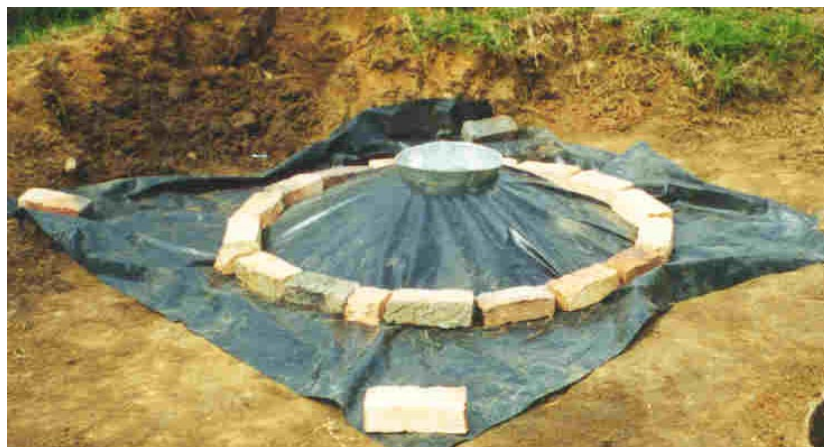
Figure 2 Mould ready for the cement render
