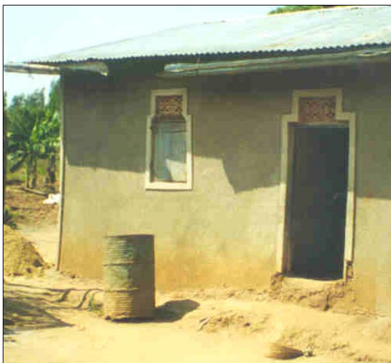
Figure 4.1: Typical informal RWH using an old 200 litre oil drum at a household in SW Uganda
