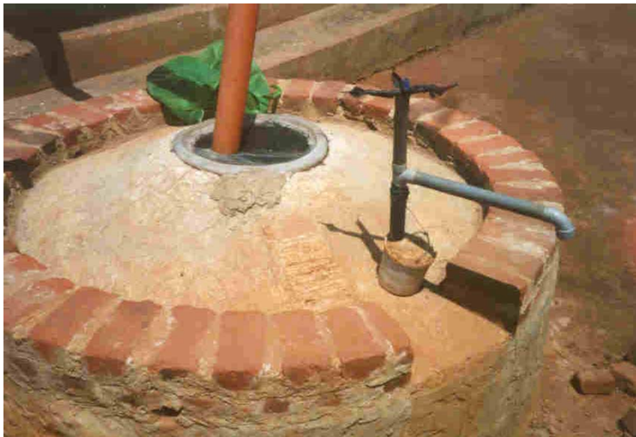
Figure 3 - A completed PBG tank showing inlet pipe and handpump for extracting water
