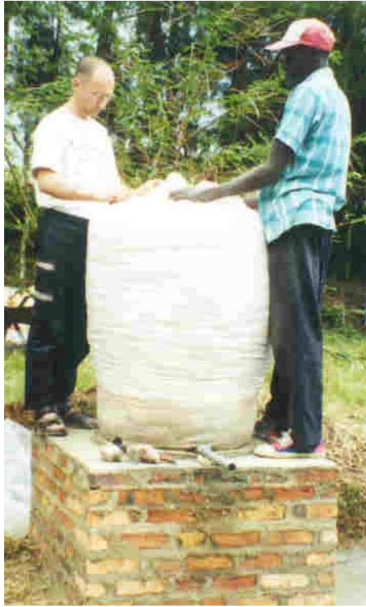
Figure 2 The filled polypropylene sack mould
