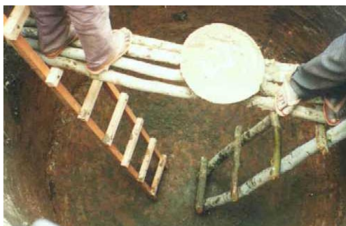
Figure 12 - Ladders and boards used to provide a working platform
