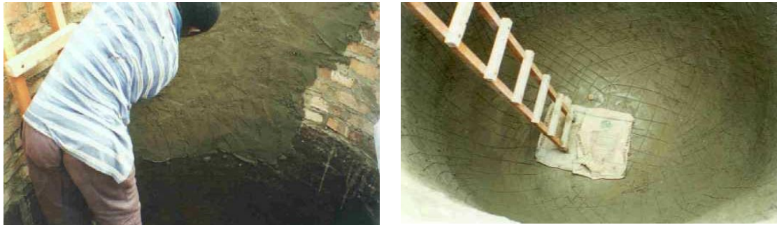
Figure 11 - showing the rendering in progress
