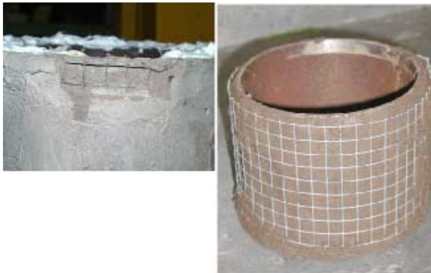
Figure 20: making a wire mesh reinforced render, (on right – applying mesh into wet mortar, on left – mortar chipped away after testing to reveal mesh).
