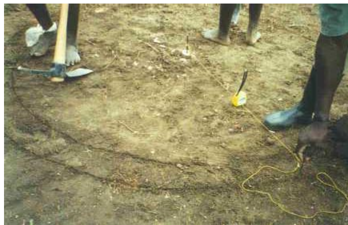
Figure 2 - Showing the cleared ground and the markings in place for the ring beam
