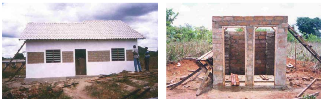
Figure 2.1 Buildings (a clinic and a latrine under construction) made from stabilised soil blocks in Tanzania
