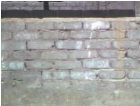
Bricks from waste material
