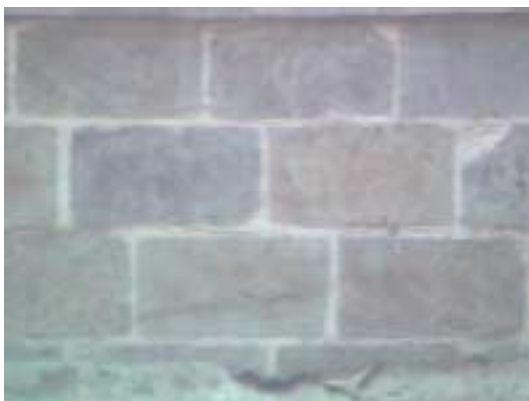
Stone cladding over bricks
