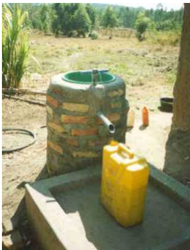
Figure 1 A 20 litre Jerrican under the Enhanced inertia handpump installed in a plastic tube tank
