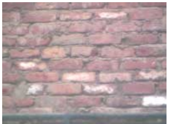
Poorly fired bricks
