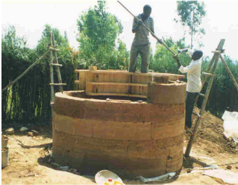
Figure 7.10 The experimental rammed earth tank under construction at Kyera Farm, Mbarara, Uganda.
