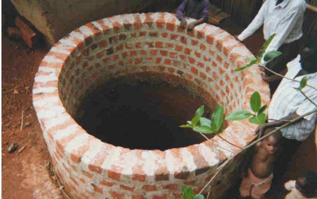
Figure 7 – Bird's eye view of the partially below-ground tank under construction.
