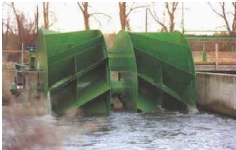
Fig. 18 (above) Photo of Staudruckmaschine installed (45)
