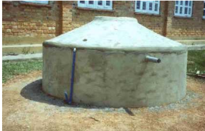
Figure 13 - The tank with cover in place
