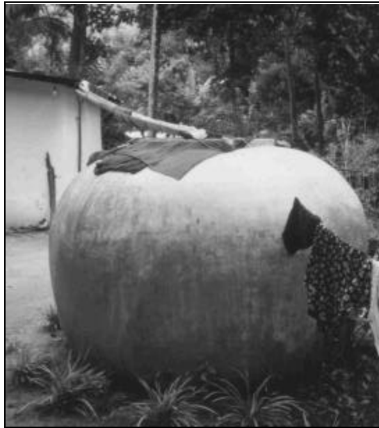
Fig. 1.1 A 8m^3 domestic ferrocement storage tank in Sri Lanka
