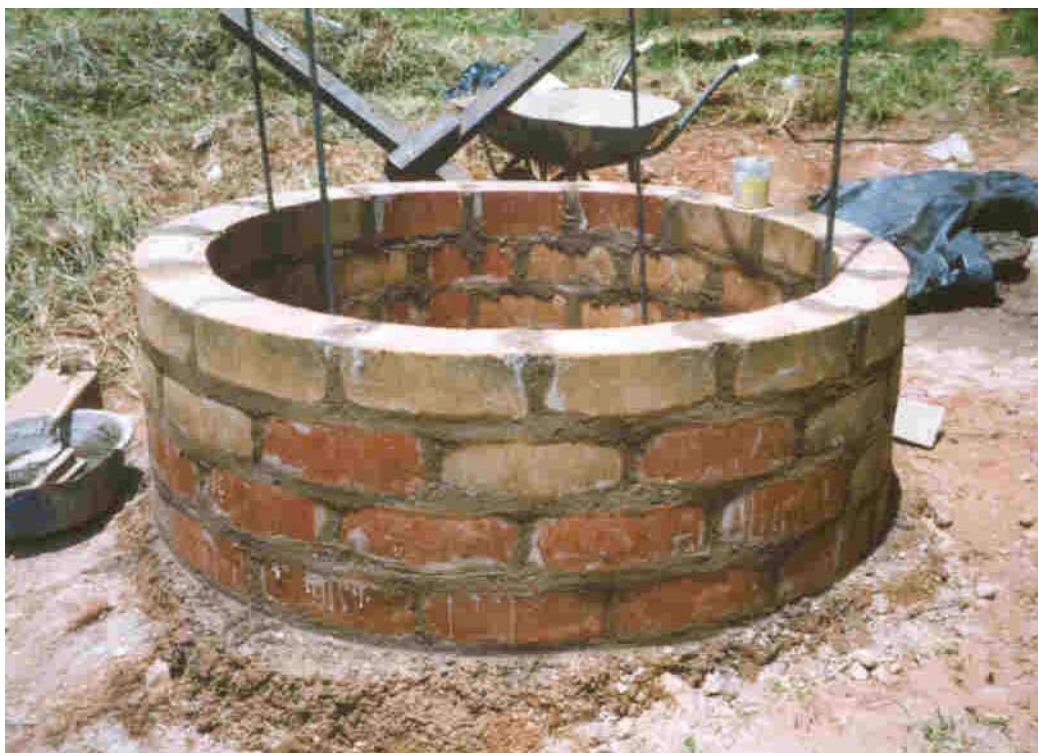
Figure 10 – Showing one of the stabilised soil block tanks under construction
