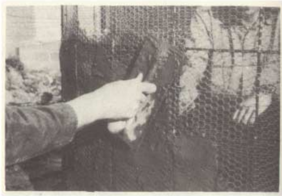
Figure 3: Construction of ferrocement tank wall (from Watt 1978)
