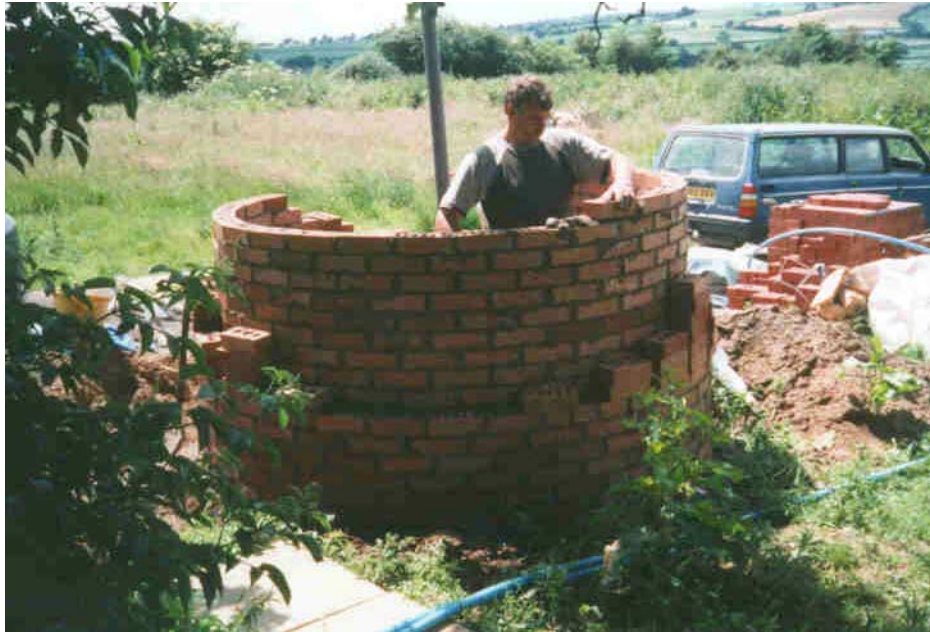
Figure 3 – Full-size experimental tank under construction at field site.
