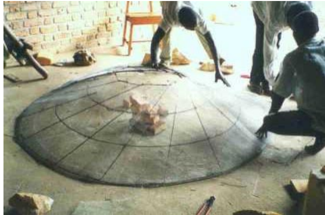
Figure 13. Applying the chicken mesh.
