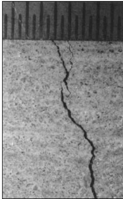
Fig. 5.21(b) Large cracks in chicken wire reinforced specimen
