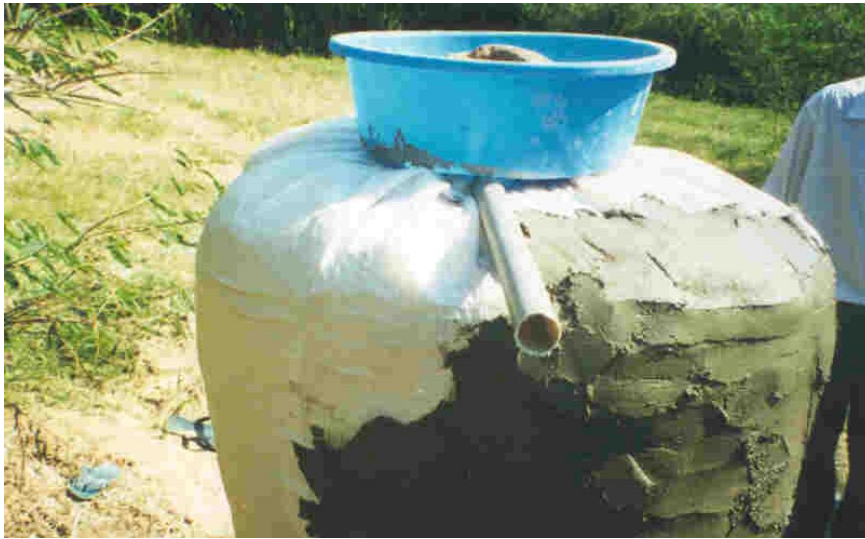
Figure 3 Overflow, filter basin and first coat application
