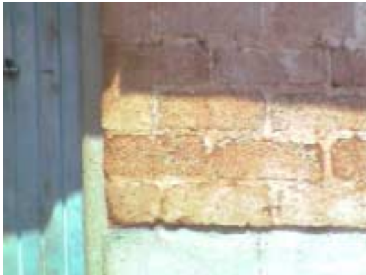
Balram block walling (self build)
