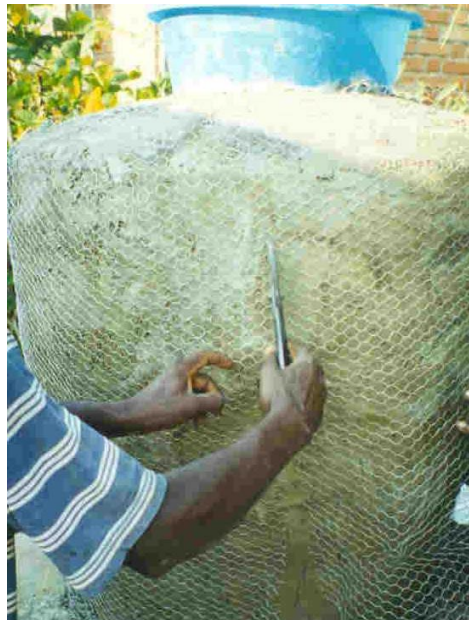
Figure 4 Applying the mesh on top of first coat
