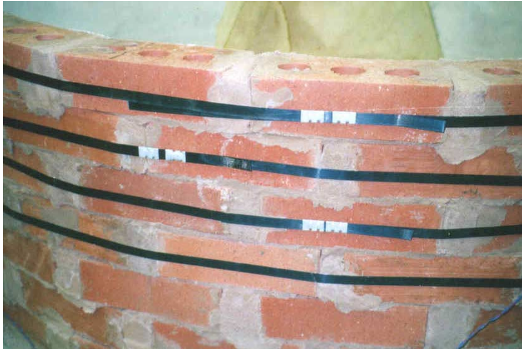
Figure 9 – photograph of straps showing crimps
