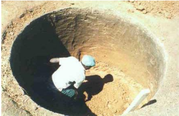
Figure 5 – Excavation of the tank
