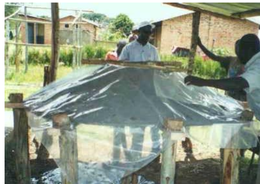
Figure 18 – Curing the cover under plastic. The cover is wetted regularly during curing.
