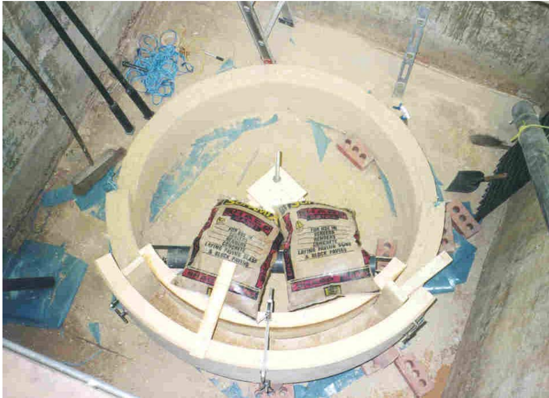
Figure 6 – Bird's eye view of the rammed earth tank under construction in the test pit at the University
