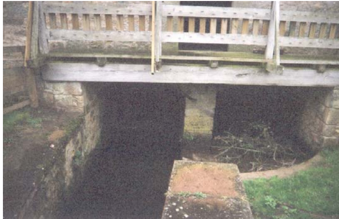
Fig. 23 Entrance to waterwheel. The rectangular inlet channel can be seen, the sluice gate is just under the wooden walkway (Authors own, 2005)
