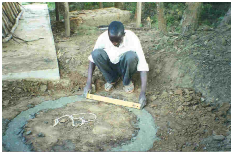
Figure 3 Checking the level of the concrete ring beam
