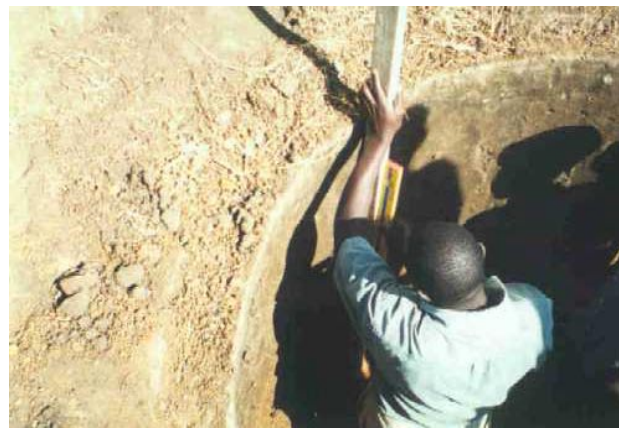
Figure 6 - Plumbing the walls to keep them vertical
