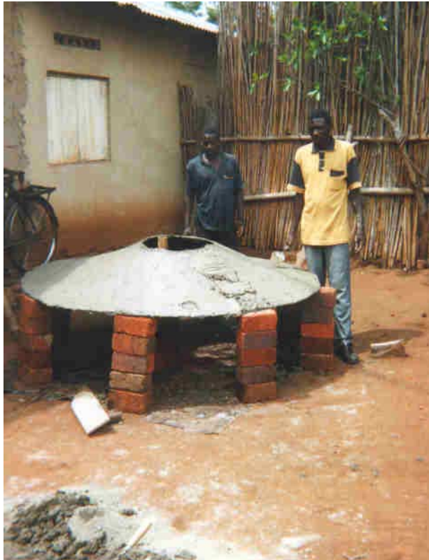
Figure 2 – A thin shell ferrocement cover near completion and ready for fitting to a PBG tank
