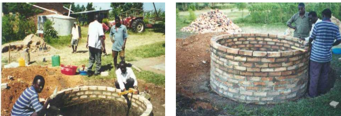
Figure 10 - showing the construction of the parapet wall
