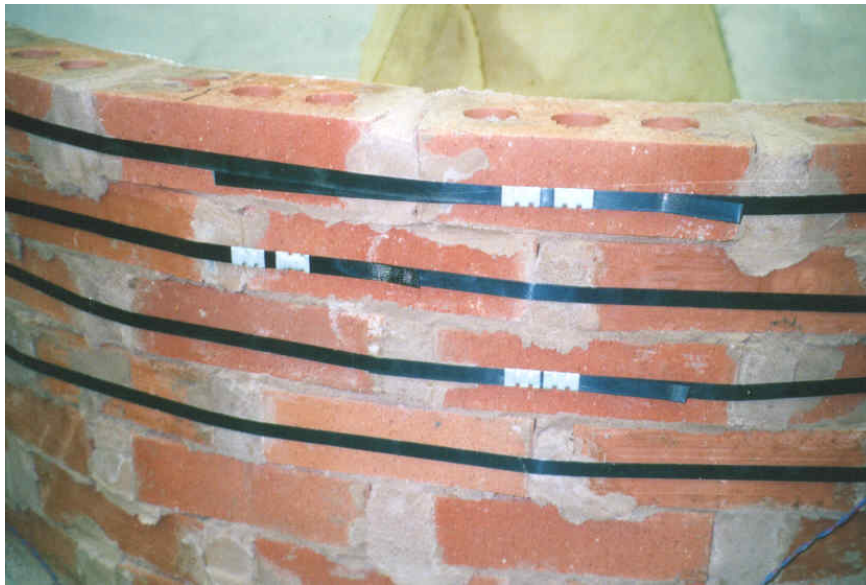
Strap showing crimps
