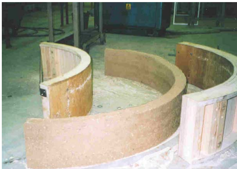
Figure 7.6 – Early experimentation with ramming wall sections
