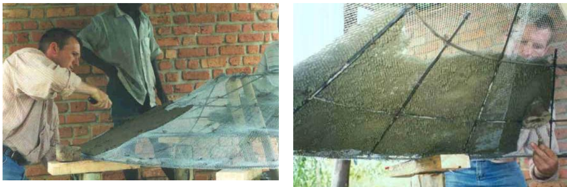
Figure 15 – applying the top coat of render to the cover
