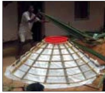
low-cost tank cover under construction
