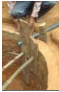
Shuttering for pump and overflow mounting
