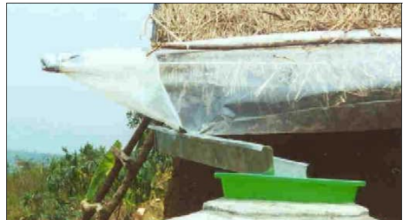
Figure 8.1: Plastic sheet guttering
