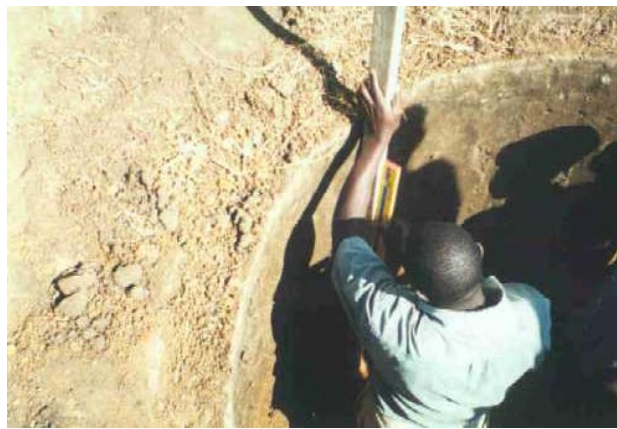
Figure 6 - Plumbing the walls to keep them vertical
