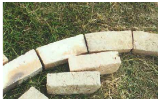
Figure 7b - The bricks with profiled ends
