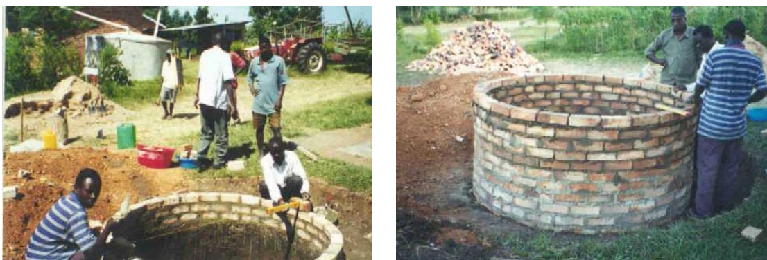
Figure 10 - showing the construction of the parapet wall
