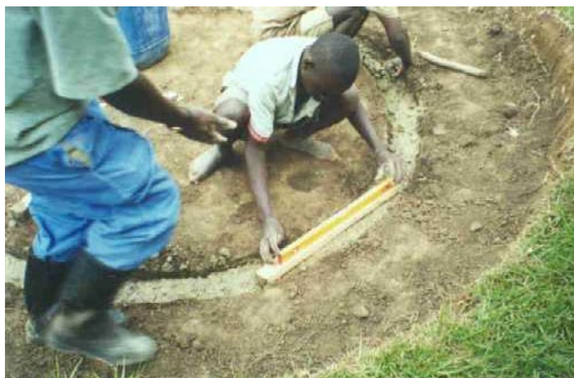
Figure 3 - Casting the ring beam
