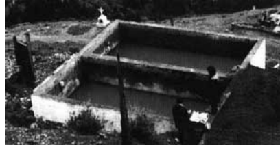
Defective Slow Sand Filter Next to the Cemetery
