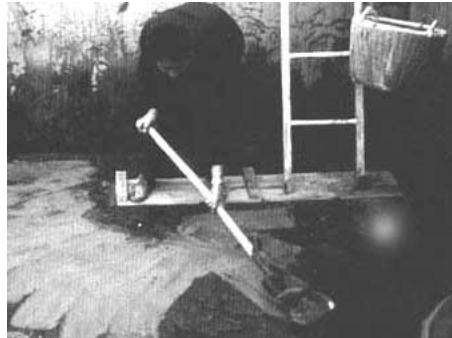
Photo 4 Cleaning of a Slow Sand Filter
