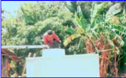
Filling the filter with filter media
