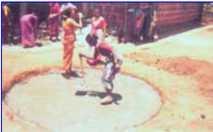
Lay the foundation
