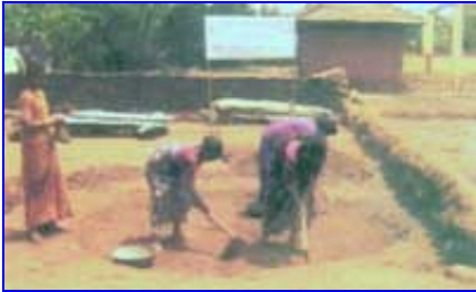
Dig to a sufficient depth to lay the foundations
