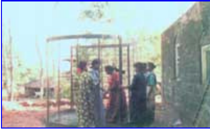
Erect the mould skeleton
