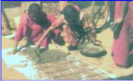
Plastering the access cover
