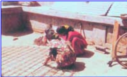
Making the cover - start with the reinforcing bars
