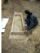
Fig. 1: This is the beginning of building the base for our frame.
