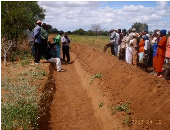
Figure 2: Complete dead level contour ready to harvest water Credit: Practical Action
