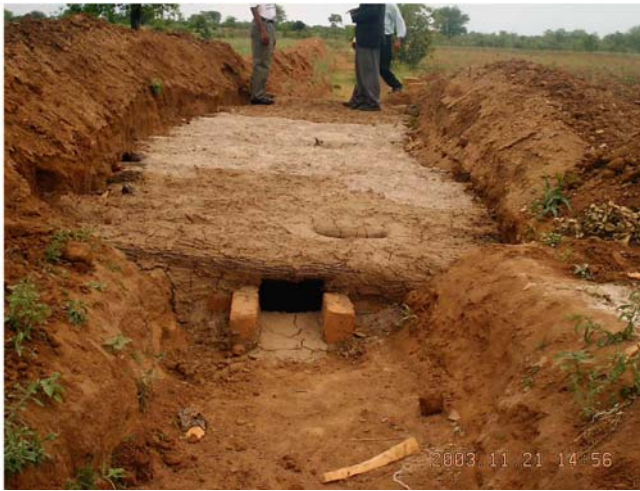
Figure 3: 10m 3 water storage facilities to avoid evaporation & deep percolation Credit: Practical Action
