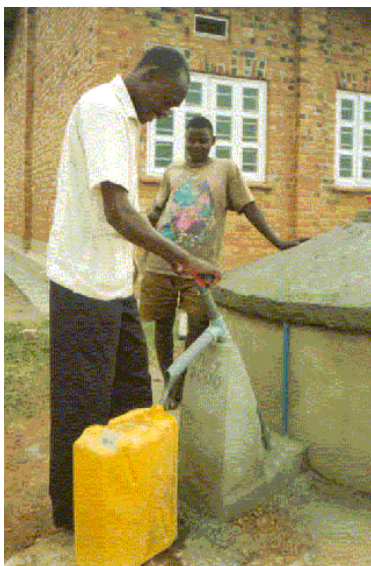
Figure 3 A Ugandan operating the Tamana handpump
