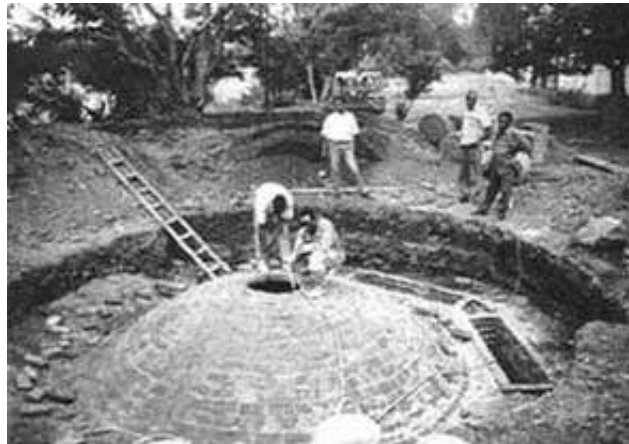
THE BIO-LATRINE INLET TOILET CHAMBERS UNDER CONSTRUCTION.
