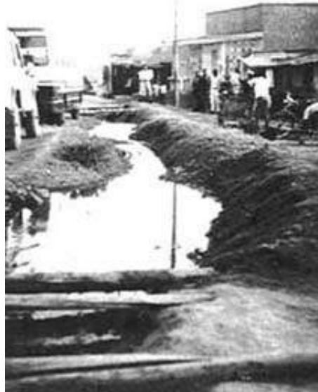
FLOOD OF WASTE WATER IN ARUSHA.
