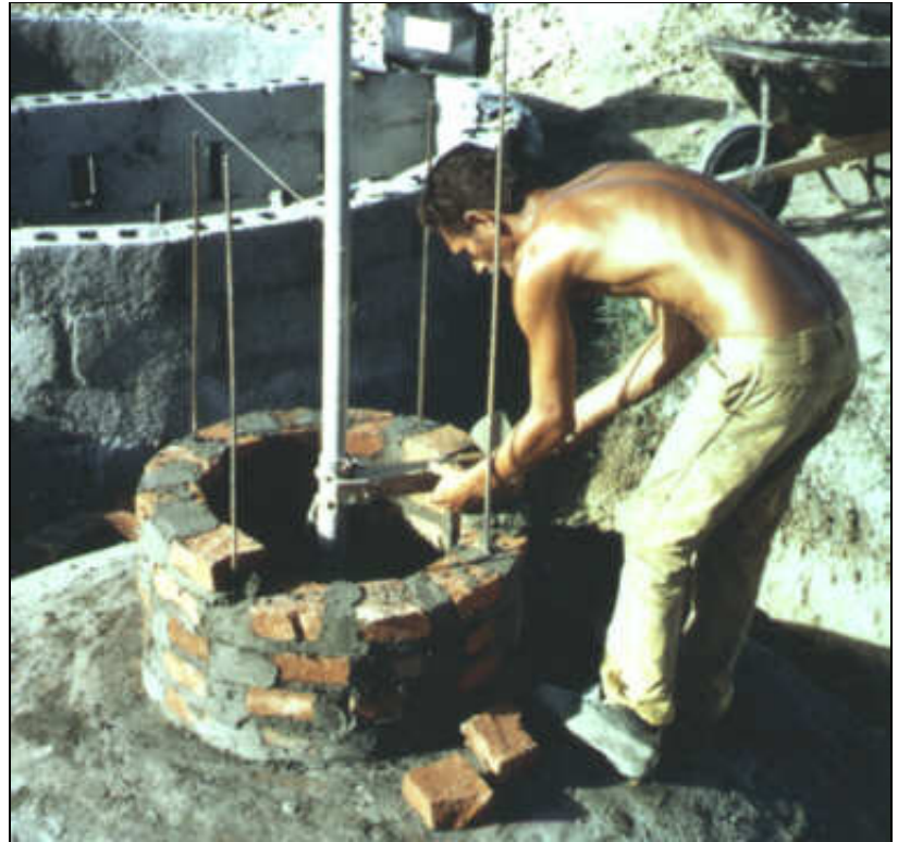
Construction of the digester neck with steel reinforcement
