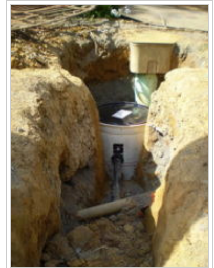
Fig 1: Sedimentation basin and pipe trench
