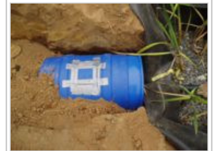
Fig 2: Surge tank and marsh inlet
