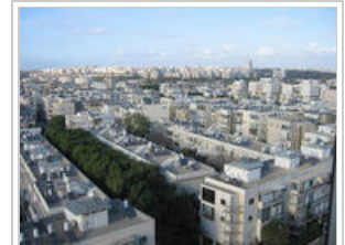
Solar hot water systems in Israel
