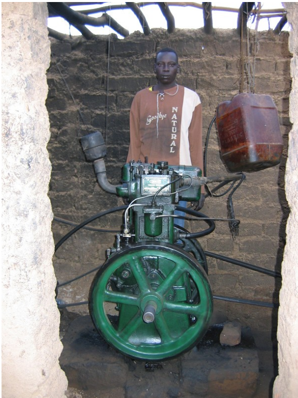
Figure 1: One of the owner's family with a diesel electricity generator in Wau Nur, Kassala. Kenya. Photo: Practical Action / Lucy Stevens.
