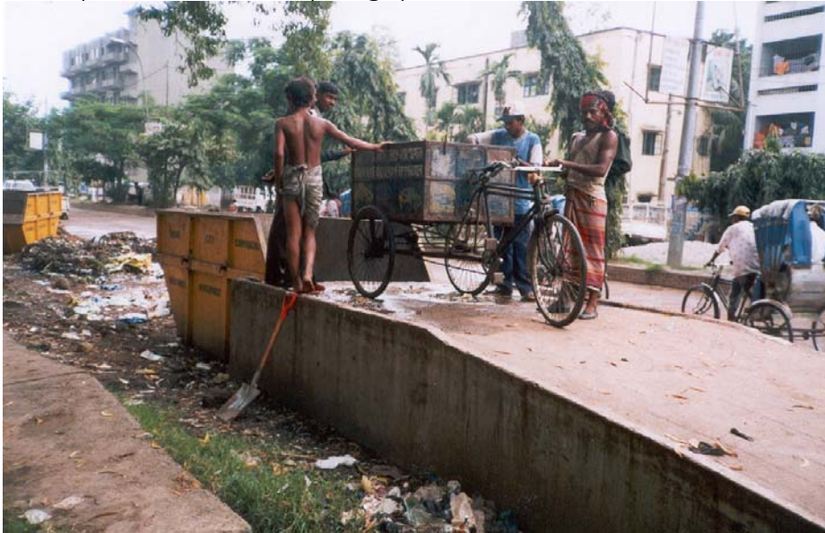
Photo 3: Ramped transfer point in Bangladesh (Jonathan Rouse)
