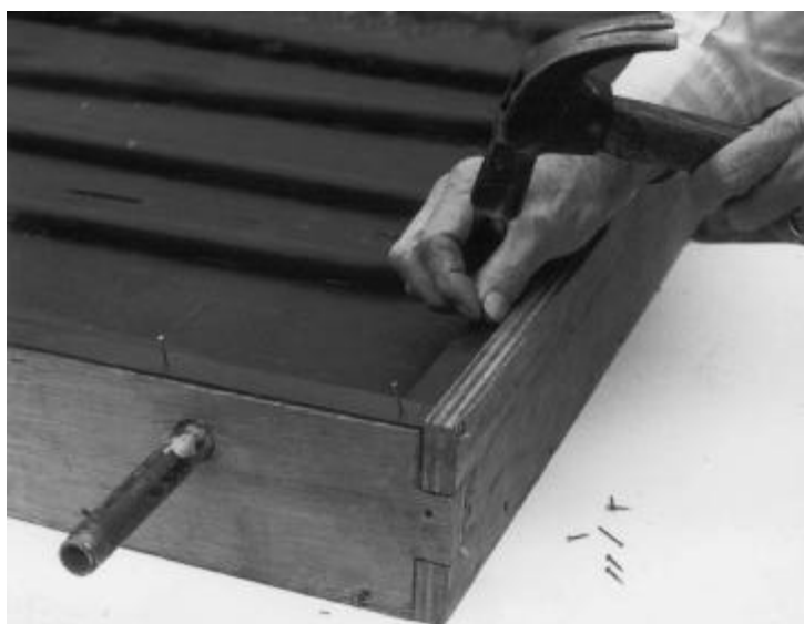
Fasten rubber strips over the rebates of sides A-B-C and D.
