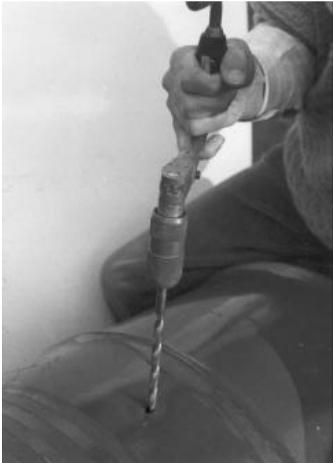
Photo 1: First, drill a hole of 6 mm and afterwards a hole of 16 mm into the marked spots.
