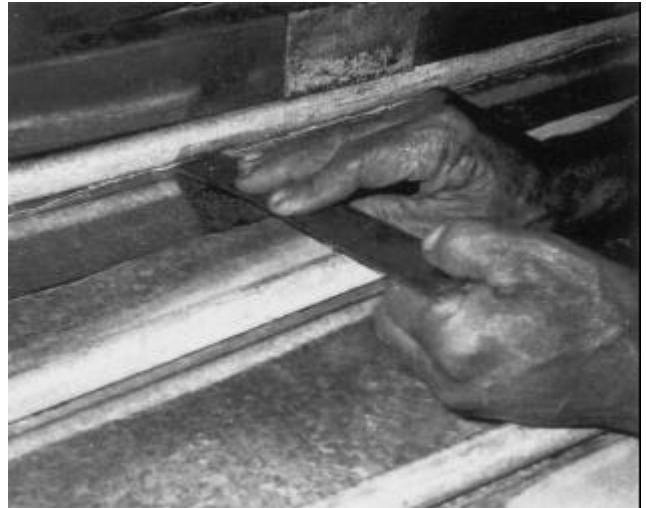
2: Press the strips firmly under the pipe.
