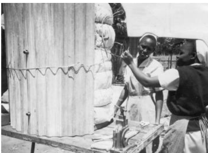
After surrounding the storage tank with insulating covers, entwine the covers with ropes or iron wire.
