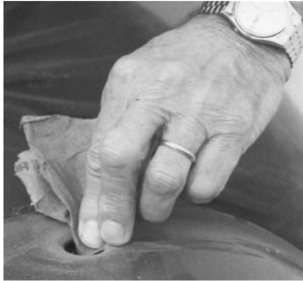
Photo 5: Thoroughly clean the pipe and driven-in hole with sand-paper.
