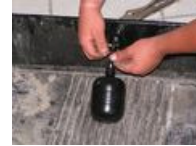
Fig 4: Installing the water basin float valve
