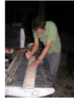
Cutting plastic for the insulation cover
