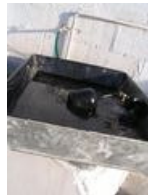
Fig 7: Water basin in action
