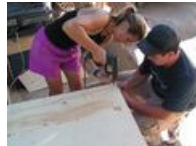
Securing the internal frame
