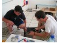
Fig 3: Drilling the intake hole for the water basin
