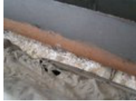
Fig 3: Sawdust may be a decent insulator but it's very messy when uncontrolled. Also encountered were styrofoam peanuts, and various loose ceramic tiles. *Materials
