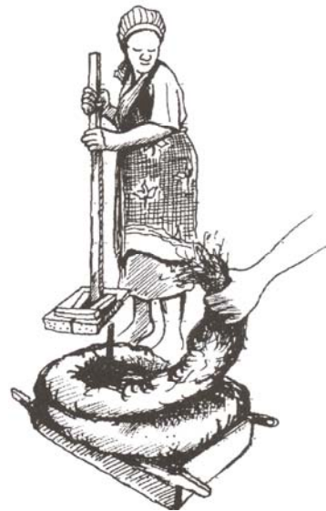
Figure 5.39 Compacting the mud rolls in the mould
