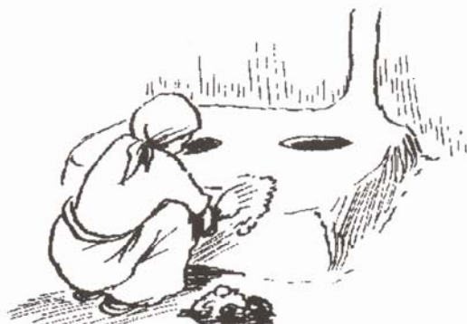
Figure A2.3 Filling in the crack with wet mud
