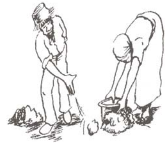
Figure 5.8 Packing mud around the sufuria
