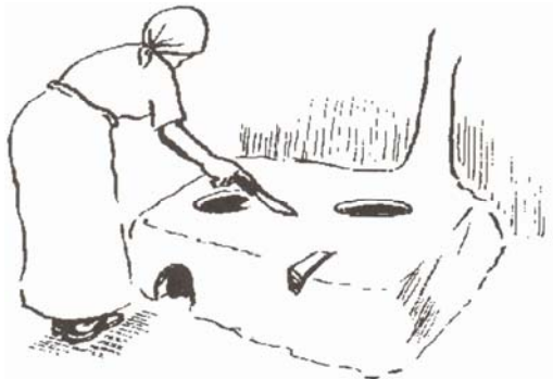
Figure A2.2 Cutting the cracked area with a knife
