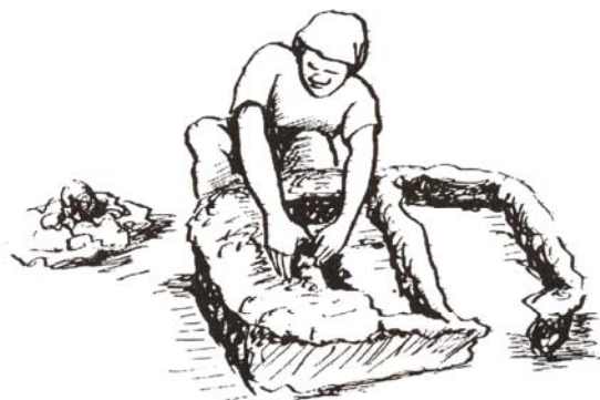
Figure 5.75 Building the top of the stove
