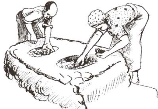
Figure 5.29 Scooping out mud to create fire chambers
