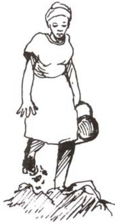
Figure 5.86 Mixing mud with water
