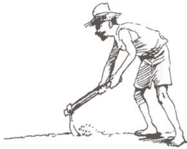
Figure 5.7 Levelling the ground
