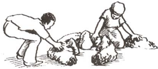
Figure 5.97 Smearing mud around the three stones
