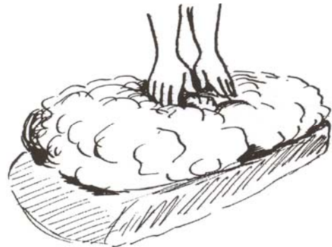
Figure 5.27 Heaping the mud balls
