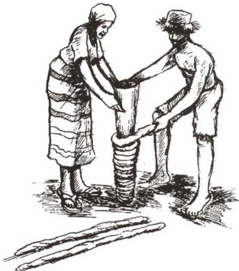
Figure A1.7 Winding the mud rolls around the stem
