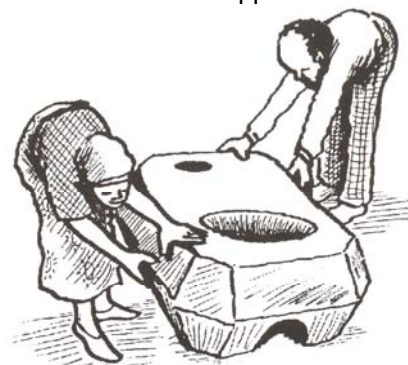
Figure 5.43 Fixing the top of the stove
