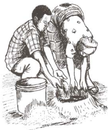
Figure 5.36 Mixing clay and sand with water
