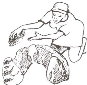
Figure 5.81 Smearing mud around the stones
