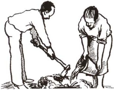
Figure 5.72 Mixing soil with water
