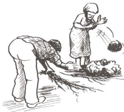
Figure 5.37 Spreading grass and throwing mud balls
