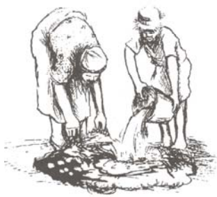
Figure 5.6 Mixing soil and water
