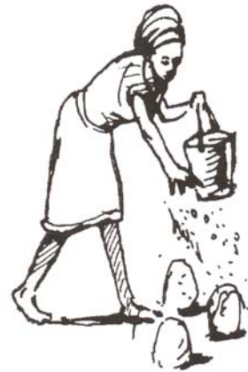
Figure 5.101 Sprinkling water on the stones
