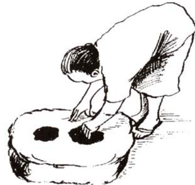
Figure 5.76 Shaping the pot holes
