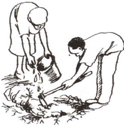
Figure 5.58 Mixing mud with water
