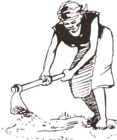
Figure 5.50 Preparing the foundations
