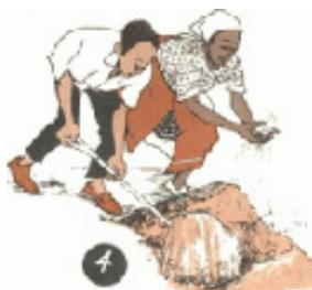
***Mix the soil and ash properly with a shovel, and then sprinkle it with handfuls of water, mixing all the time, just like making cement. The best way to do this is to have one person turning the soil, and the other throwing on the water.***
