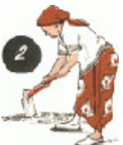
**Level the floor where you are going to put your jiko, and sprinkle it with water to make it damp but not muddy.**
