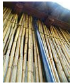
Pipe for gases created from decomposition to escape out back
