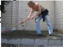
Fig.1b The section of dirt under the concrete blocks was compacted with a base plate tamper.
