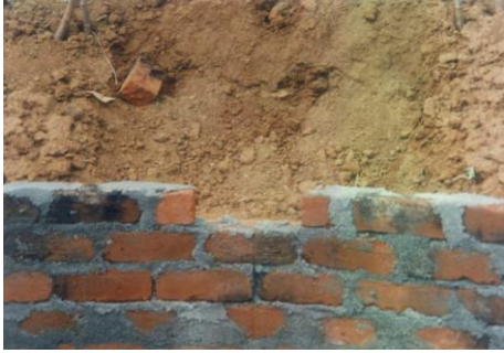
Figure 10: Outlet of the tank
