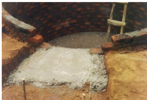
Figure 7: Concrete base for the inlet construction
