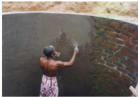
Figure 12: Plastering the tank
