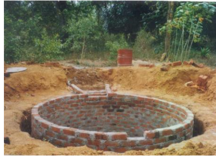
Figure 11: Completed tank before plastering
