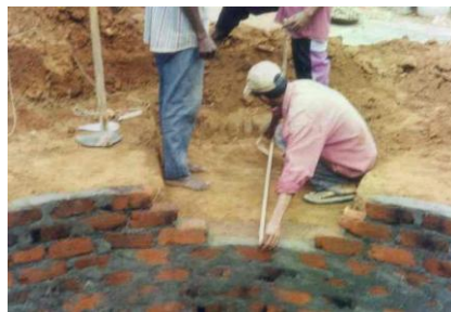
Figure 6: Measurement taken for the inlet construction
