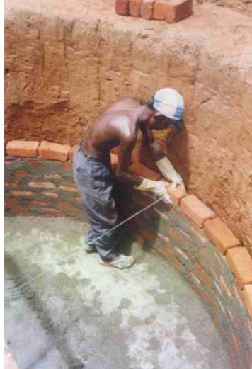
Figure 5: Wall construction of the tank on the concrete base
