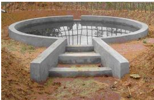
Figure 14: After the completion of the rainwater-harvesting tank
