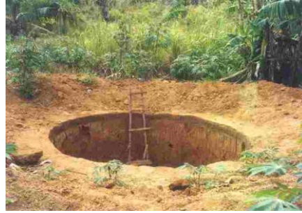
Figure 3: Pit for the tank construction
