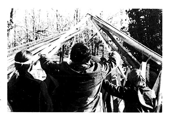
To equalize weight distribution during roof assembly, you might have to switch to the opposite side of your yurt and begin roof assembly there.
