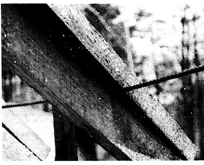
Sandwiching the cable between roof pieces; nail above the cable itself.
