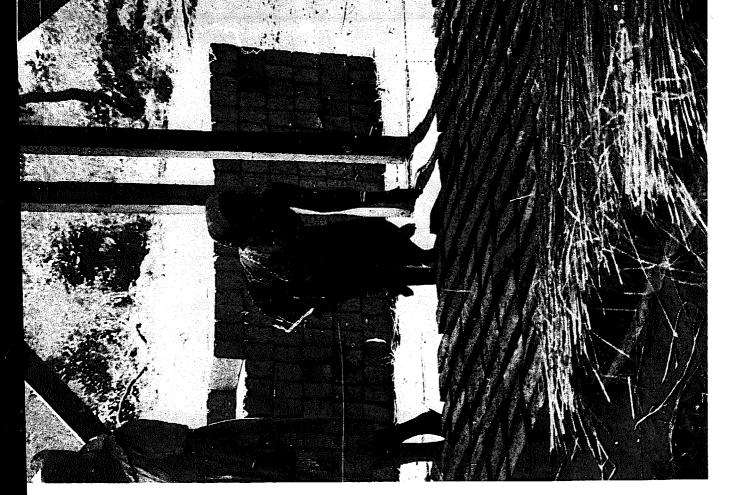
Pressed bricks were allowed to cure for two weeks before going into the walls.
