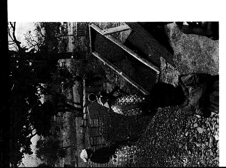
Sieving separated the fine earth for brick-making from the coarse material that was used to fill in under the floor.
