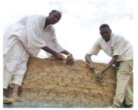
**Pic 16.** The wire mesh is tied around the partly made dome
