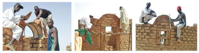
**Pic 8.** Building the window arch using a metal girder
