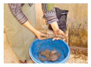
**Pic 1**. The mud should be mixed with water to form a sticky substance
