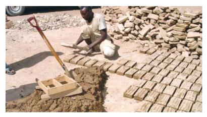
Pic 4. A participant using a moulding cast for brick production
