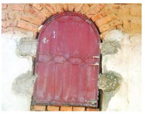
**Pic 27.** Cement is used to fix the window frame in place
