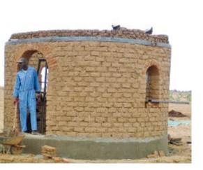
**Pic 14.** Bricks are laid for the formation of the dome
