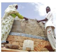
**Pic 17.** Cement is plastered on top of the wire mesh
