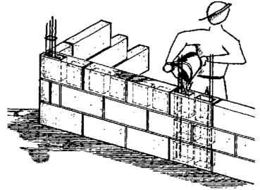
Figure 36: Filling the corners with concrete and reinforcing bars
