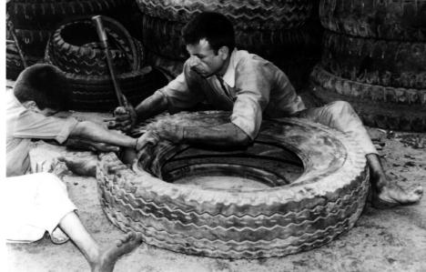
Figure 2: Manual Separation of the Tread from the Sidewalls, Karachi, Pakistan Photo: PCSIR – WASTE
