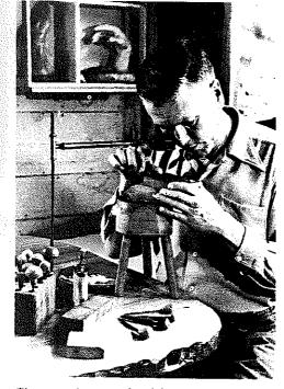
The engraving reproduced here was engraved on endgrain wood, using traditional burins. The burin's flat upright allows it to slide along the thumb during the tool's cutting strokes.
