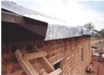
Splash-guard being nailed into a roof
