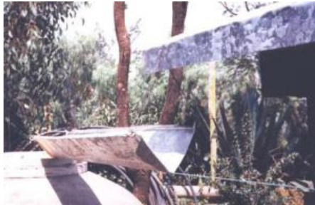
The first gutter laid along a drawn string
