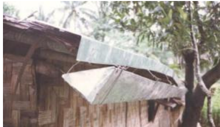
Gutters fitted into hangers tied to a splash-guard nailed onto an uneven roof
