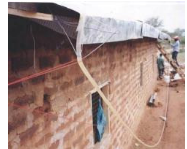
Water level in a hosepipe filled with water
