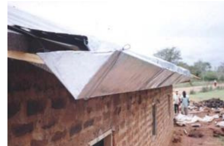
Gutter laid in hangers
