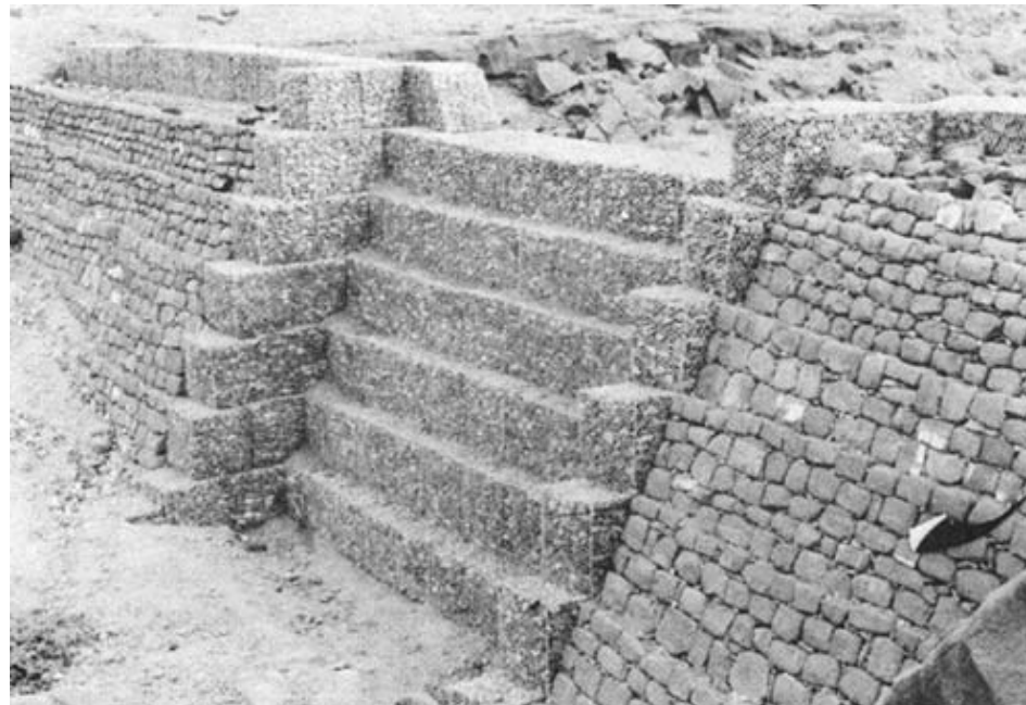
Weir made from gabions and dry-stone work (Cape Verde)
