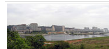
The Malaysian government Ministry of Finance building in Putrajaya.
