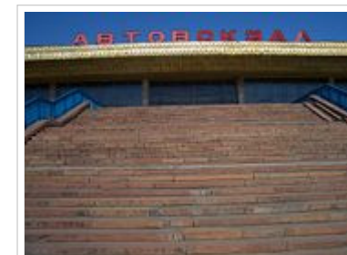
Bishkek West Bus Terminal
