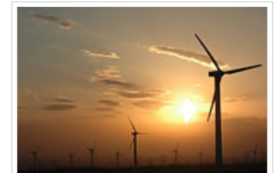
Windmill generators in Xinjiang. The Dabancheng project is Asia's largest wind power plant.
