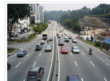
The Damansara Link section of Klang Valley's Sprint Expressway.
