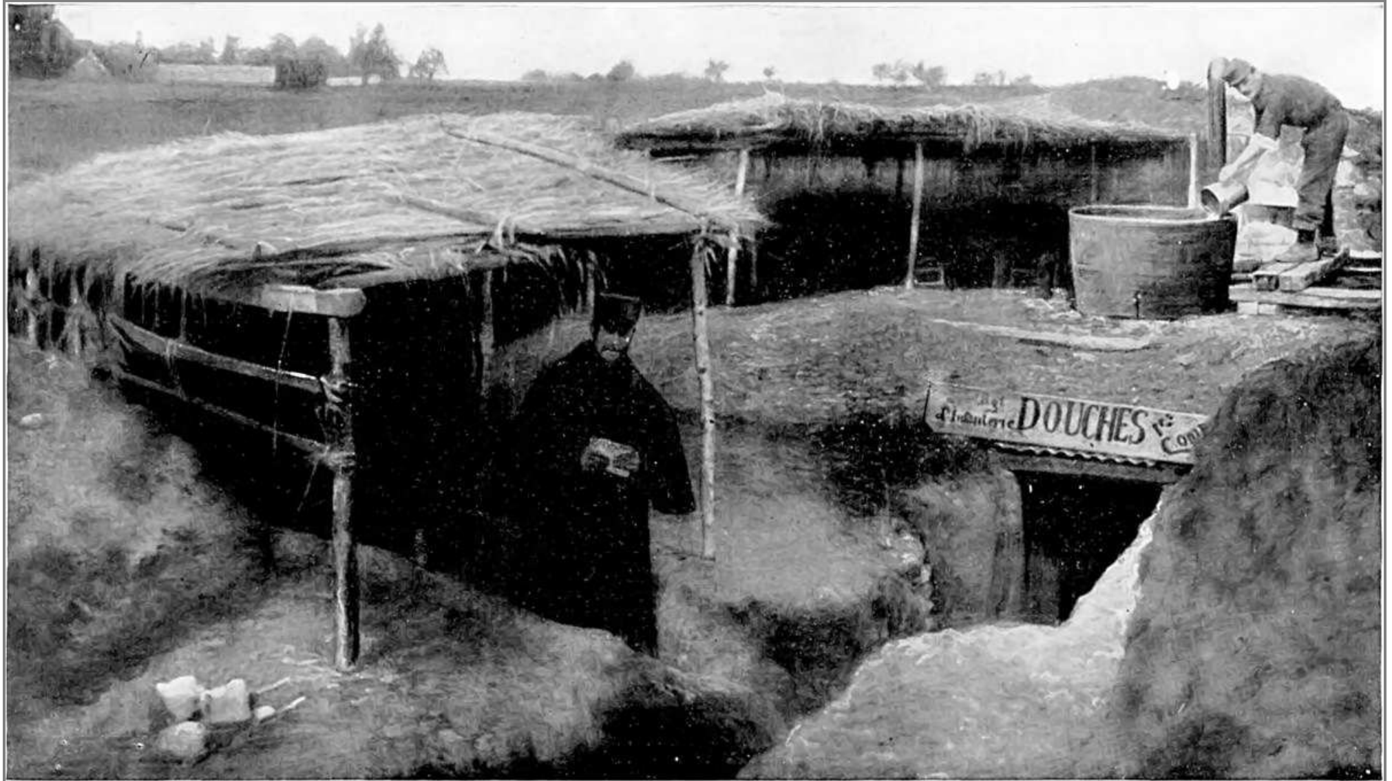
SYBARITISM IN THE TRENCHES! A HOT SHOWER-BATH ESTABLISHMENT INSTALLED BY AN INGENUOUS FRENCH ENGINEER.
